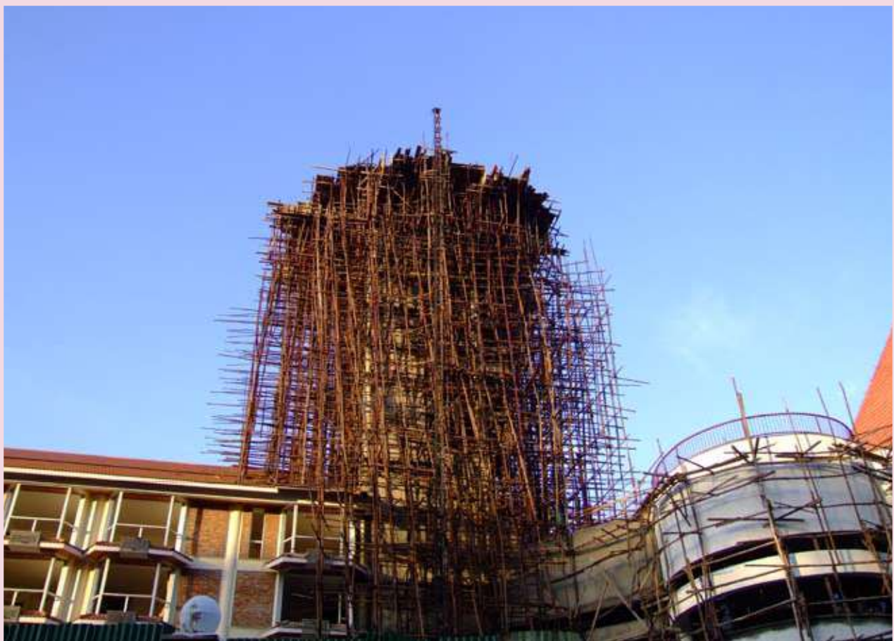
Eucalyptus scaffolding poles supporting Kampala's developing economy.
